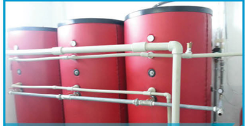
Installation of hot water tanks/boilers in series
