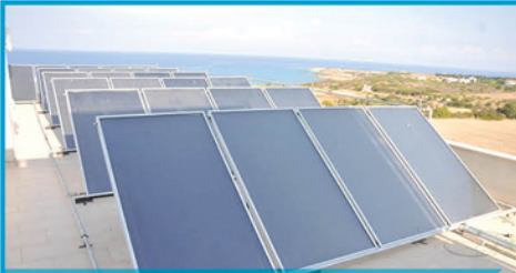
Installation of selective surface solar collectors
